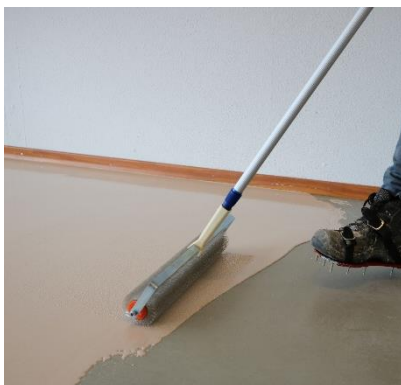
Roll with spiked roller to remove surface tension.
