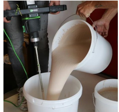
Pour blended mixture into clean bucket.
