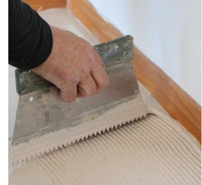
Trowel on, material self-levels.
