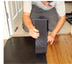
LVT Installation on InstaLay Peel & Stick Underlay
