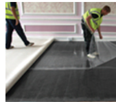
Carpet Installation on InstaLay Peel & Stick Underlay
